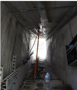
Inclinometer casing being slid through the gallery
