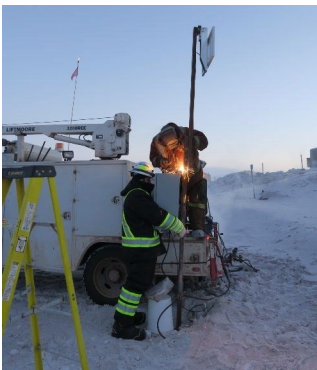
Installation of the casing and solar panel
