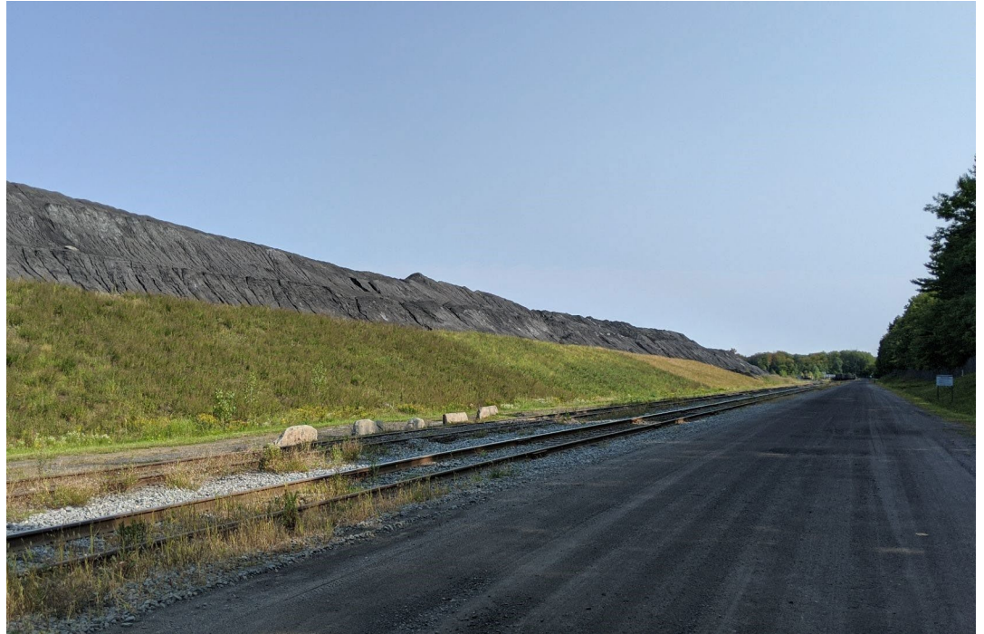
Rio Tinto Fer et Titane (RTFT) P84 dry tailings located in Québec | Partially remediated active TSF dry stack
