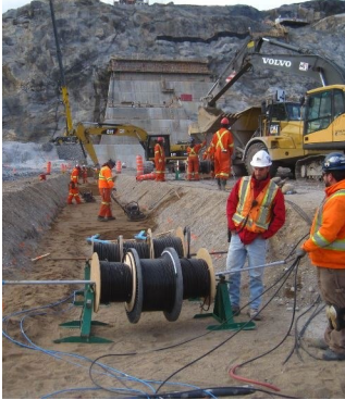
Installation 4500HD piezometers.
