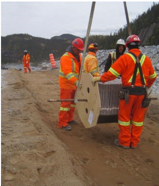
Upstream Horizontal SAAS Installation.
