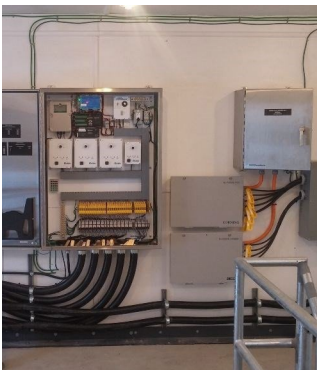
Custom DL Series Dataloggers, Hydro Quebec standards.
