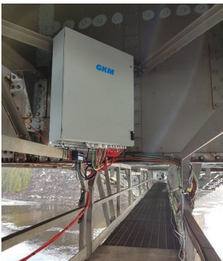
One of the two custom-made data acquisition systems installed under the Alexandra bridge.
