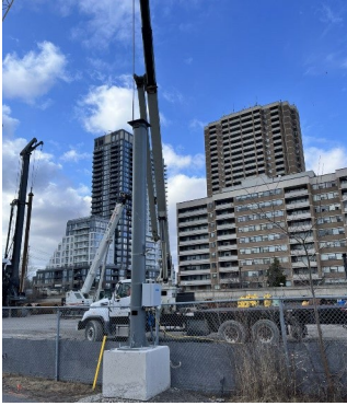
Gravity base installation
