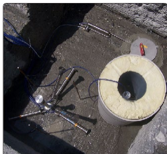
◆ Instrumentation cluster in dam body
