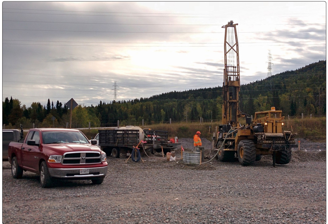
Piezometer installation in geotechnical boreholes
