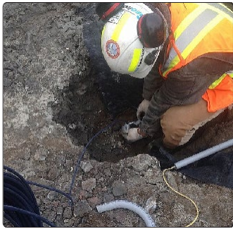
◆ Shape Accel Array (SAA) installation in vertical orientation
