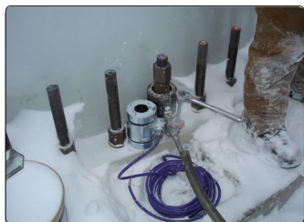
◆ Load cells installation on anchors
