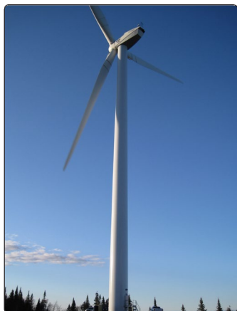
◆ 80 meter T-2 Wind turbine view
