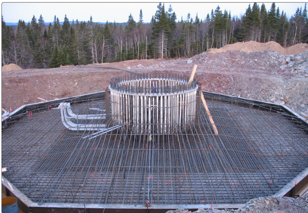
Foundation steel pad reinforcement, anchors and tower instrumentation
