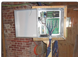
◆ Automated data acquisition system for telemetry
