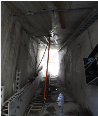
Inclinometer casing being slid through the gallery
