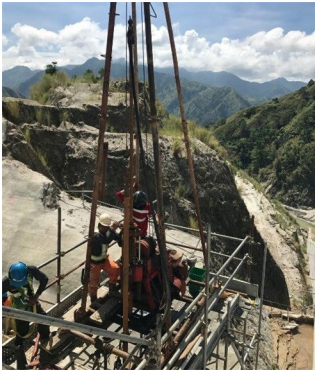
Borehole drilling for extensometer installation
