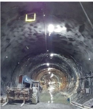
Instrumented shotcrete tunnel liner section
