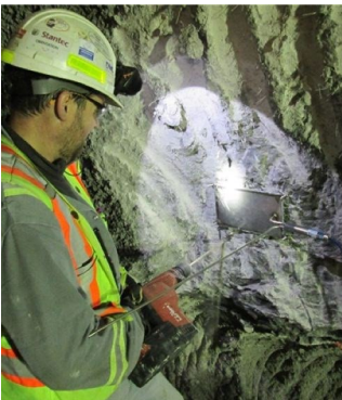
NATM pressure cells installed at the interface of the shotcrete tunnel liner and natural ground
