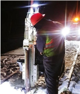
Drilling with Geoprobe Rig
