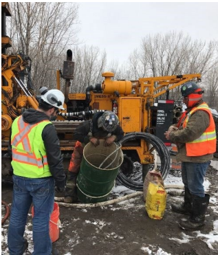
Preparation of grout
