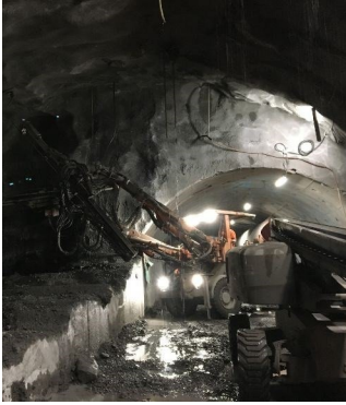
Installation of extensometers in the tunnel
