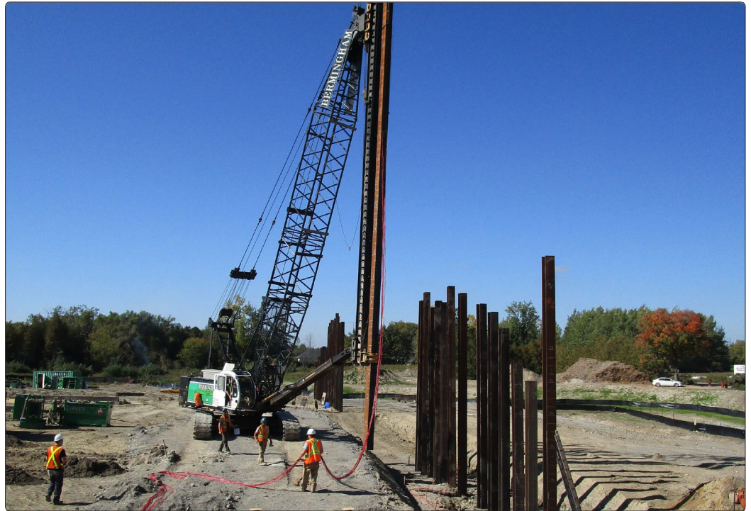
Instrumented pile being maneuvered into position
