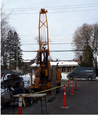
Drilling and installation of multi-point extensometers
