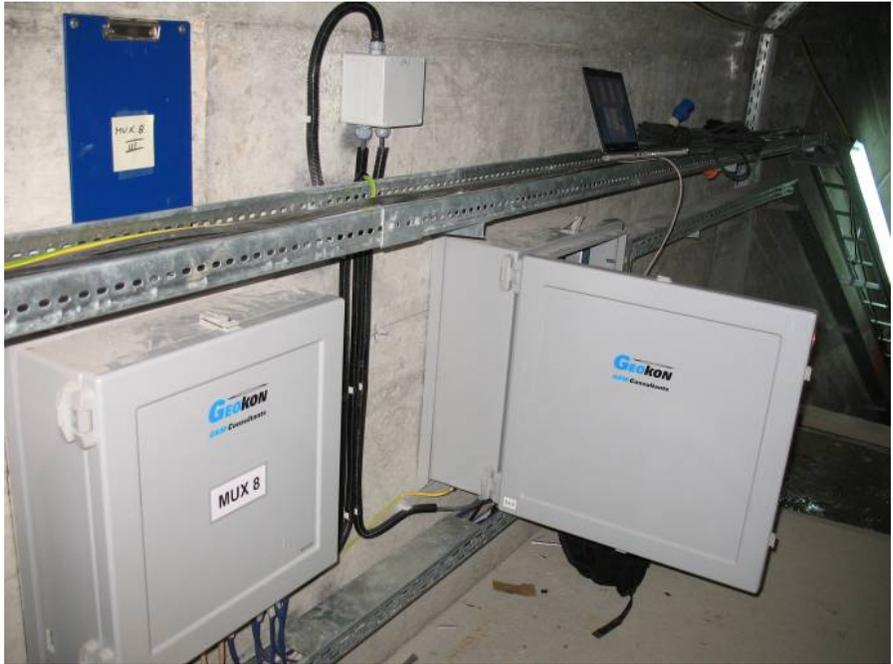
Figure 8: Typical secondary station and multiplexer installation
